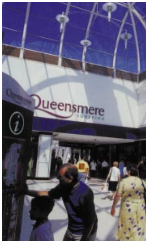
Figure 4 Alders Square showing new domed roof and pendant lighting
