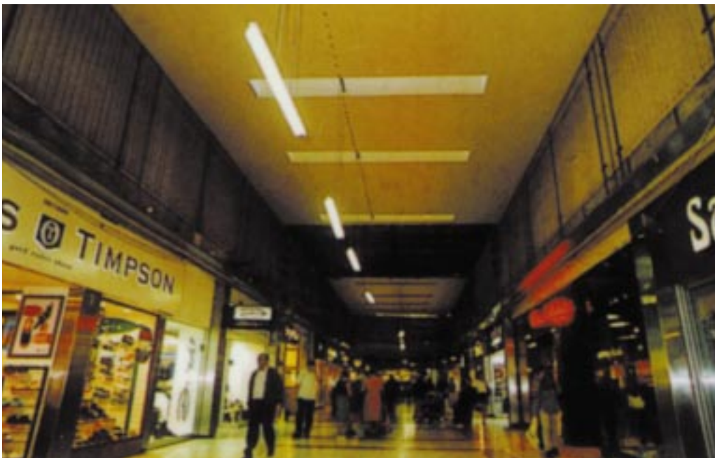
Figure 5 Curzon Mall during refurbishment
