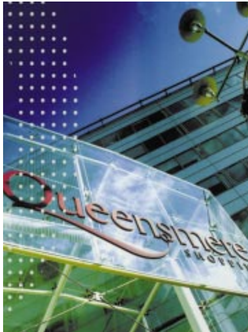
Figure 11 New glazed canopy over main entrance to the Centre
