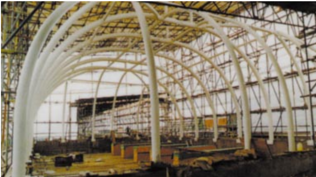
Figure 1 Construction of new domed roof during refurbishment
